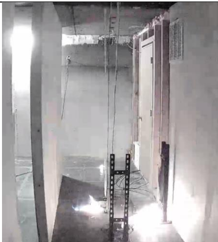
Ignition of the refrigerant 12s after refrigerant release.
