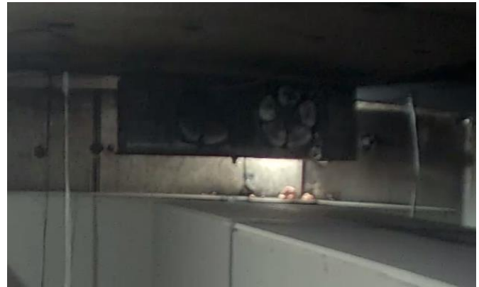
After the discharge was completed the fan stopped rotation and the frost began to melt away.
